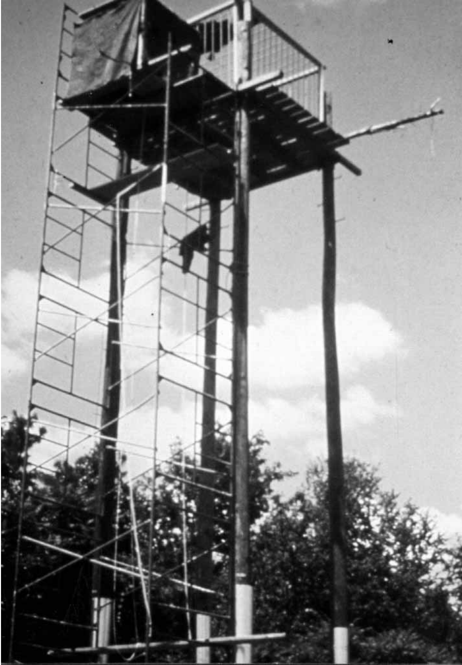
This hacking tower, located in New York, allows a commanding view by the eaglet(s) and security from predators. The adjacent scaffolding houses the feeding platform and blind. Photo by Peter Nye.
